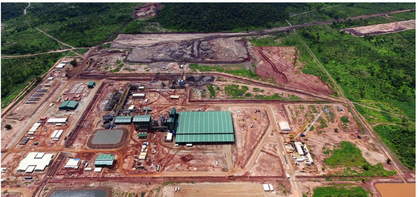
FIGURE 2. AREAL PHOTO OF A GRAPHITE MINE IN NORTHERN MOZAMBIQUE
